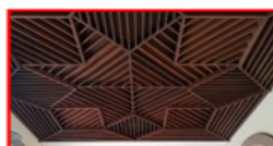
Ceiling of Islamic Center
